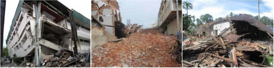
Fig. 12. Three major damage classifications in Padang, damage on reinforced concrete building (left), damage on nonreinforced concrete (center), and damage on ordinary residential houses (right).
