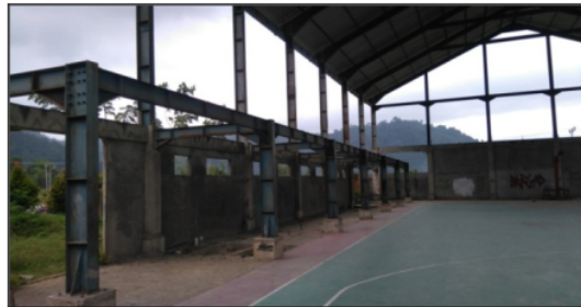
(a) The view from inside the hall building
