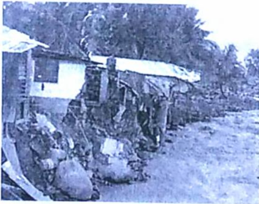
Figure 1. Scouring on the the river bang of Batang Kuranji due galodo I
