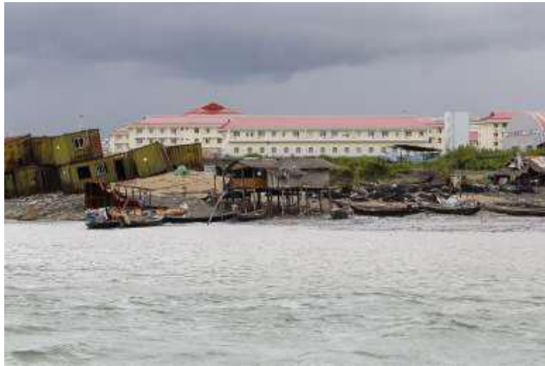
Figure 3: Damage to Resident's Houses
