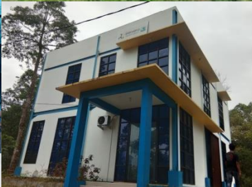
RESERVOIR KAP. 20 M3
