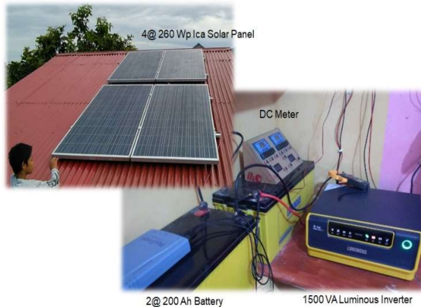
Fig. 2. Residential rooftop PV system 1000 kW
