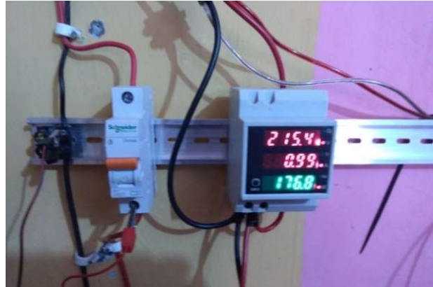
Fig. 3. AC bus measurement PV off-grid output for various loads
