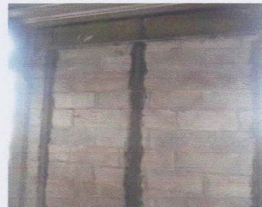
Fig. 17 : Construction of walls at core area
