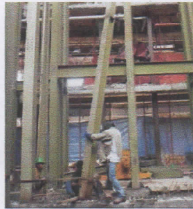
Fig. 13 : Erection of steel construction in the core area
