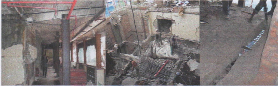
Fig. 10 : Temporary support using H profiles
