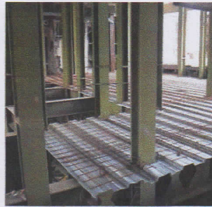
Fig. 14 : Slab at core area
