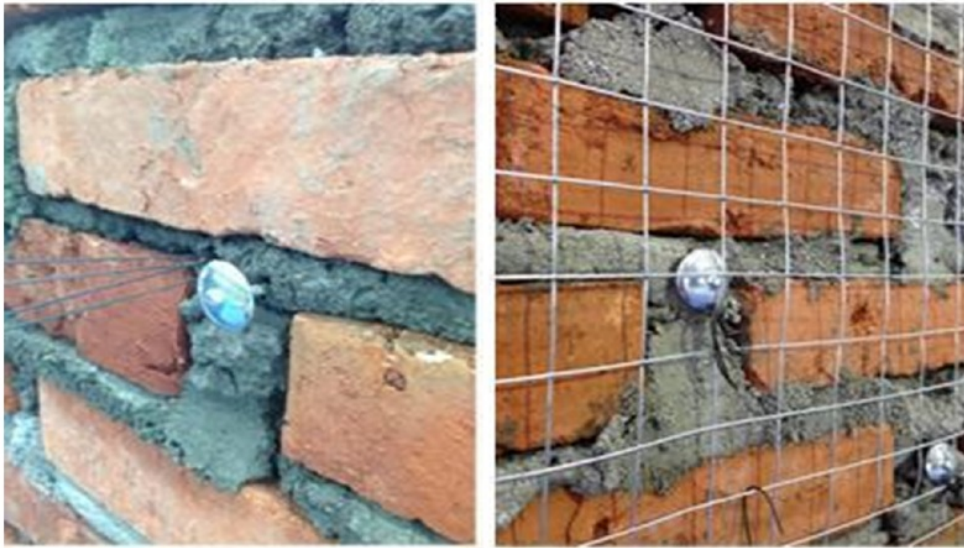
Figure 6 Detail of attach of the wire-mesh
