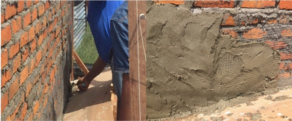
Figure 8 Construction and plastering the wire-mesh
