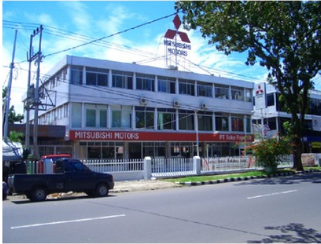
Photo 2. Collapsed Building before the 2007 Earthquakes
