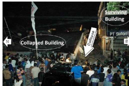
Photo 1. Collapsed and Moderately Damaged Buildings Due to the 2007 Sumatra, Indonesia Earthquakes (Source: Padang Ekspres Newspaper)
