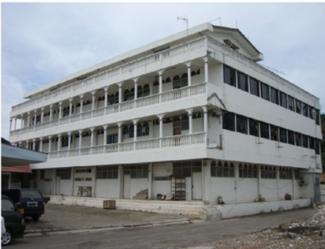
Photo 3. Surviving Building after the 2007 Earthquakes
