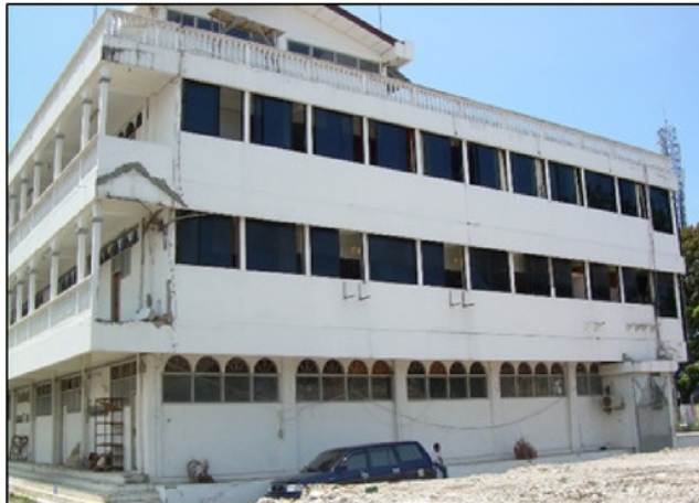
Figure 1 Surviving R/C frame building suffered sumatera earthquake 2007 [6]
