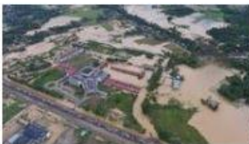
Figure 2. Top view of government office center in Air Pacah
